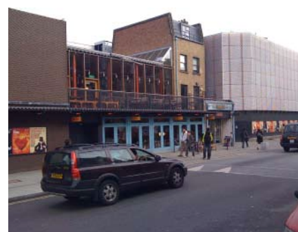
Above Example of how an existing building, such as a pub or bar, may be retained and incorporated as part of a new mixed use development.
